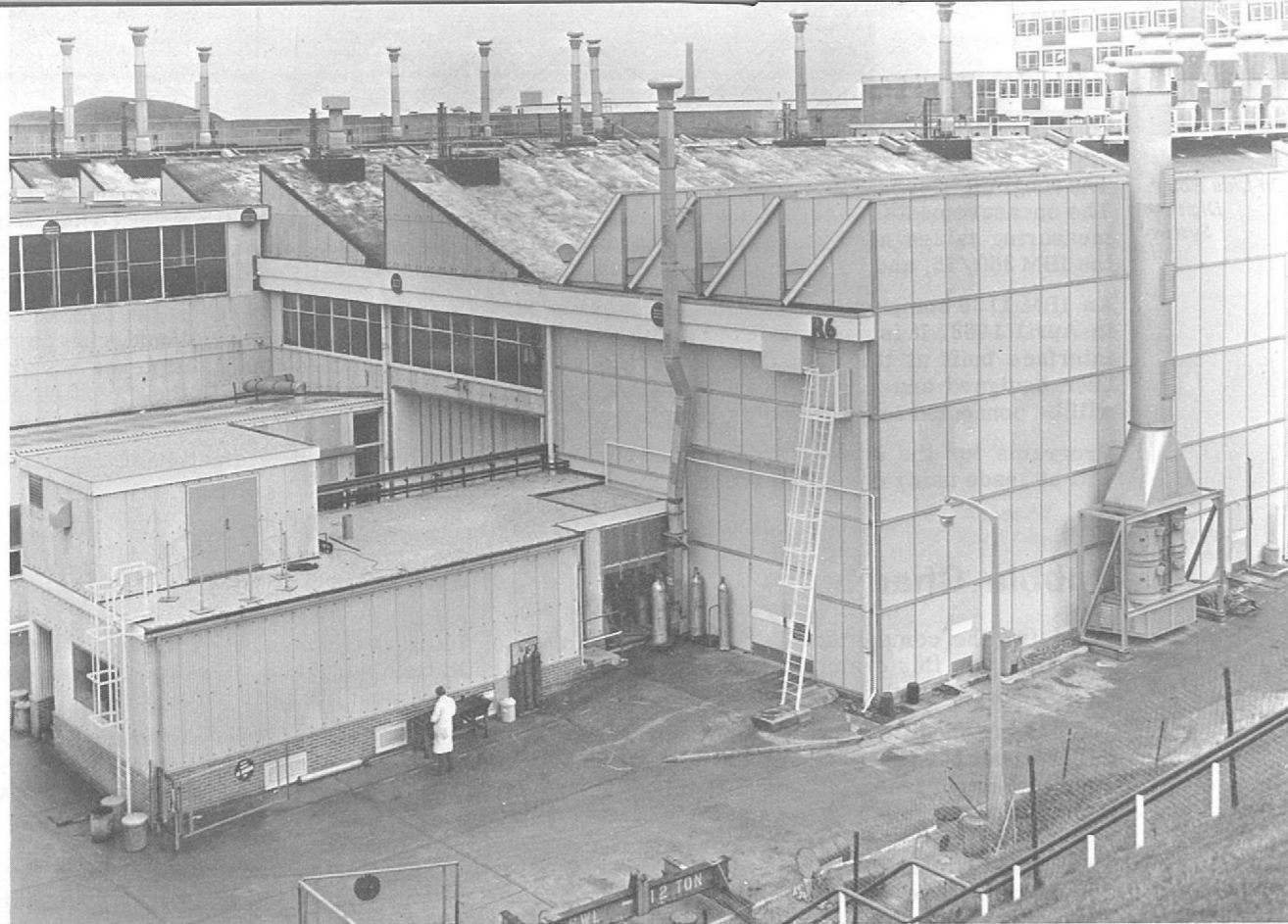
Figure 59. Heavy Liquid Bubble Chamber Building modified for use with propane — showing separate control room, expanded polystyrene frangible walls and extract ventilation plant.
