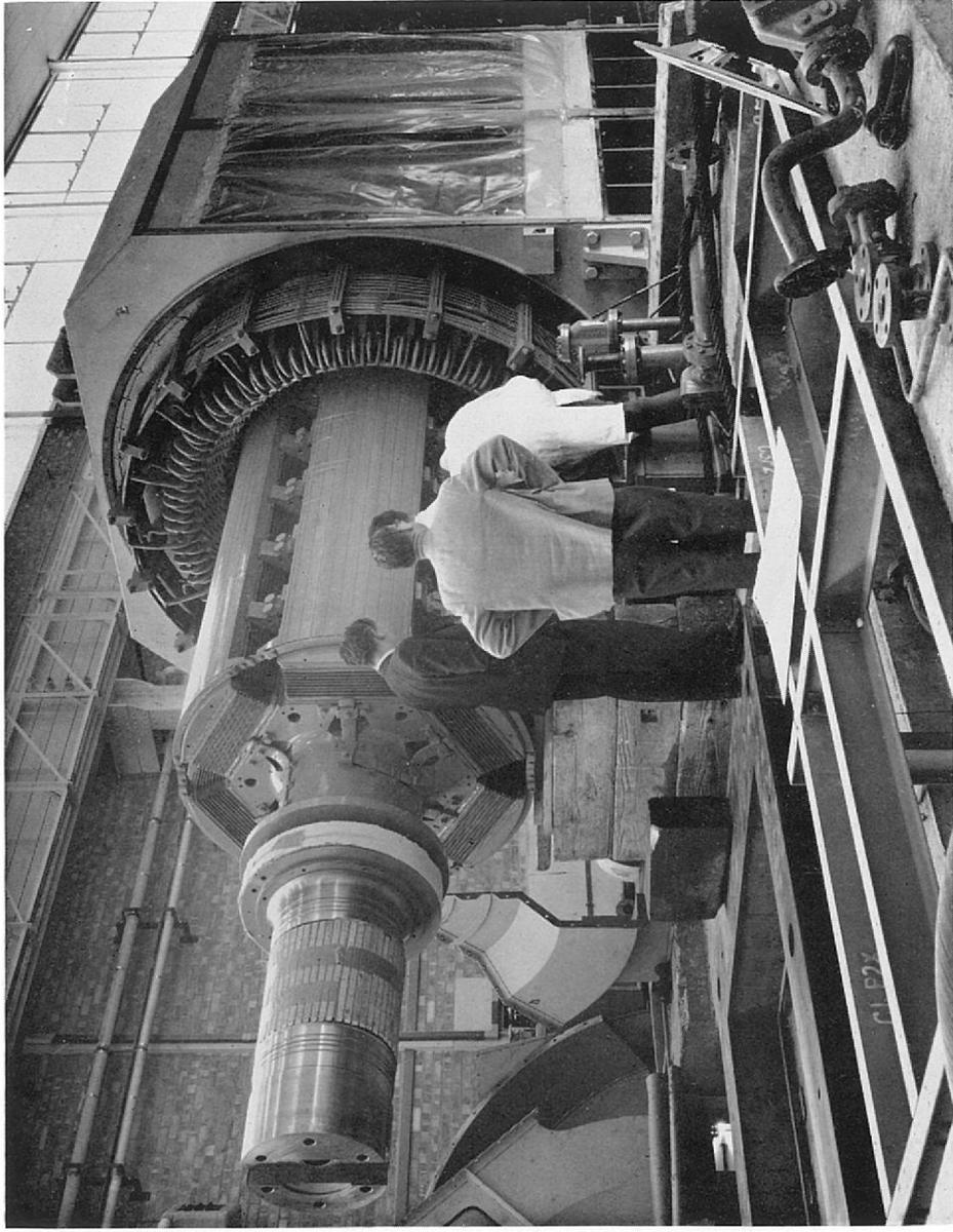
Assembly of alternator for Nimrod Power Supplies.
