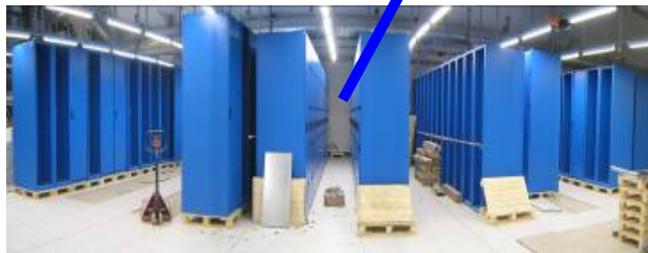
Electronics "Counting" Room(s) Trigger Systems. DAQ Systems.
